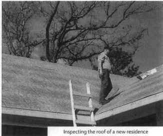
Inspecting the roof of a new residence
