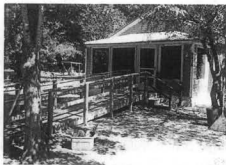
Home Repair Program: Wheelchair Ramp built
