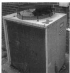
Admin Building SOE
